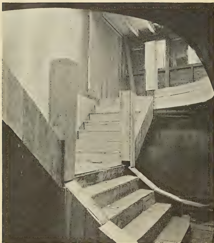
( Photograph by Morse Dry Dock & Repair Company ) Fig. 10.—Stairway Under Construction
